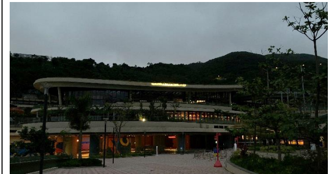
OP06 Responsive Lighting Design – General view of lighting design with appropriate level of lighting to reduce potential impact
